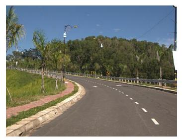
one, two or more lanes arranged within a single carriageway with no median (divider) to separate opposing flows of traffic.
